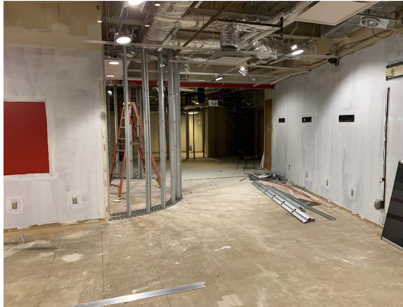
Progress Photo – October 2021
