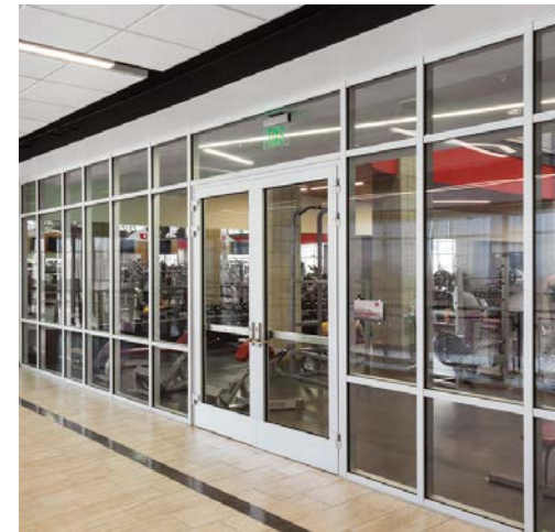
4 Storefront: Aluminum and Glass door and partitions
